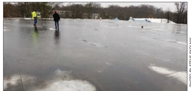
Roofing contractors gaze over the lake of standing water on the roof of the Co-op on January 24.
